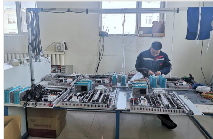
ELECTRICAL APPLIANCE CABINET
