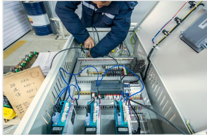
MAIN CONTROL BOX ASSEMBLY
