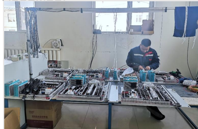
ELECTRICAL APPLIANCE CABINET
