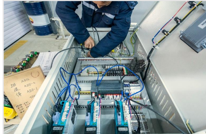
MAIN CONTROL BOX ASSEMBLY
